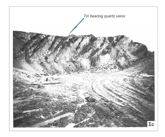
Plate 2: 1950's photo of the Abbaretz pit wall looking west showing south dipping tin-bearing veins (dark grey)
